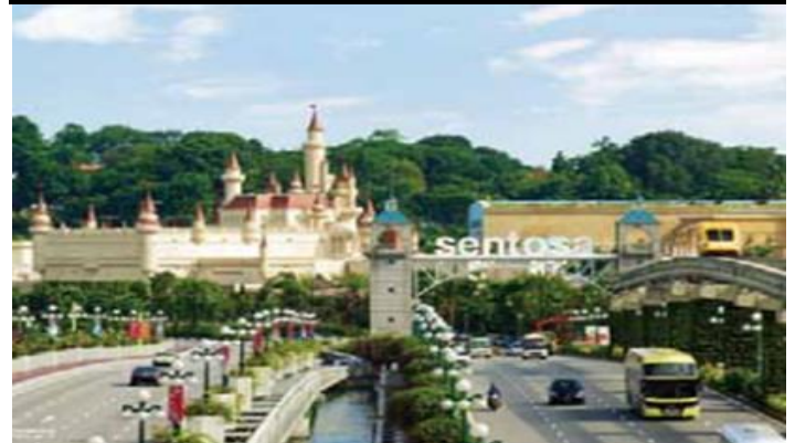
Figure 34: Sentosa second vehicular bridge
