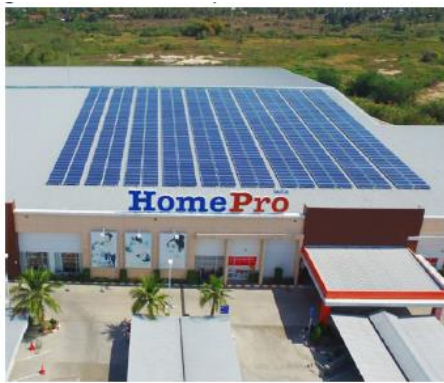
Figure 3: Reduce carbon emissions by installing solar panels in stores
