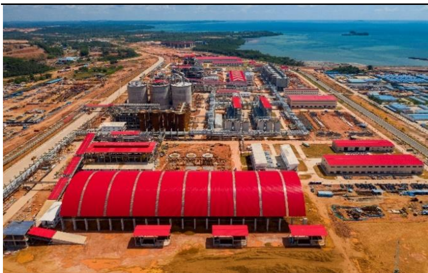
Fig 7: PT Bintan Alumina refinery
