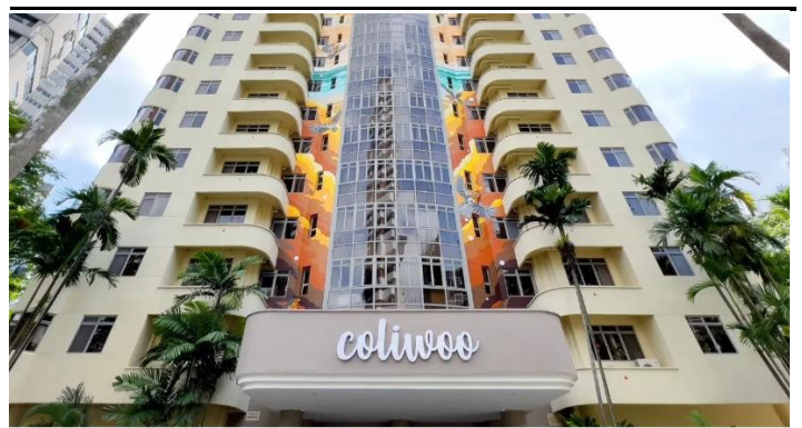
Fig 15: Main building of Coliwoo Orchard
