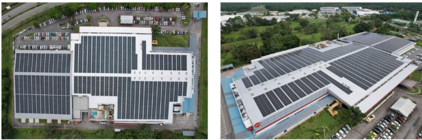
Figure 2: Rooftop solar installed on P1-P3
