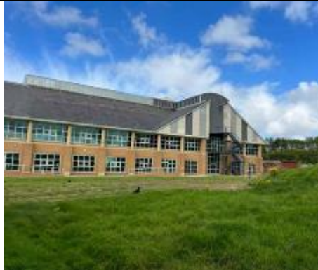
Fig 15: Peel Park consists of two buildings used as a back office
