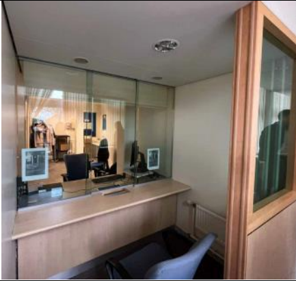
Fig 3: A JCP with reinforced area for claimants who may present threats to the centre staff
