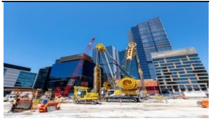
Figure 11: Ground view of Parramatta metro station
