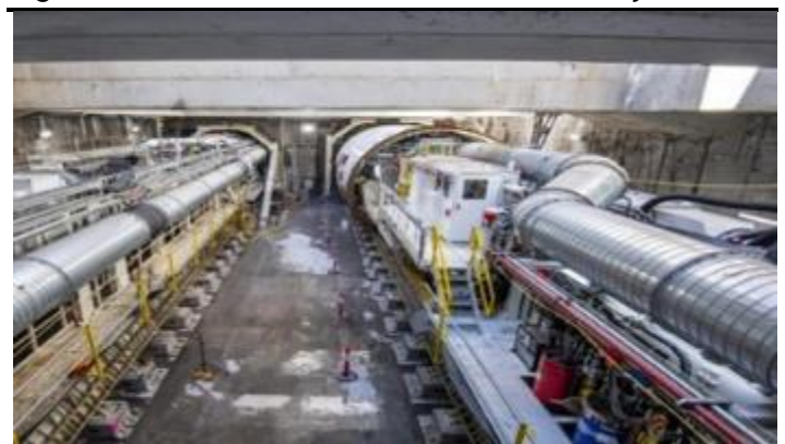
Figure 13: Ground view of Rosehill Services Facility
