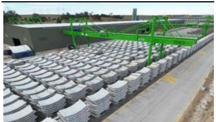
Figure 15: Ground view of Eastern Creek Precast Facility
