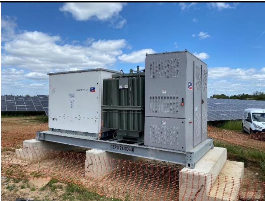
Fig 8: Bunkers Hill - inverter substation
