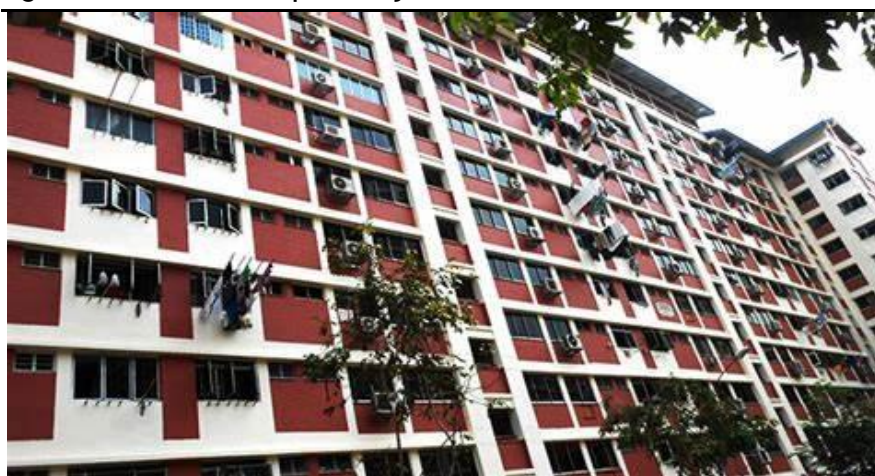
Fig 2: Bishan Street 22 Repaint Project
