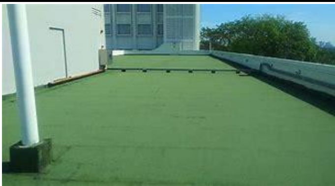
Fig 15: Green Label waterproofing membrane at NUS
