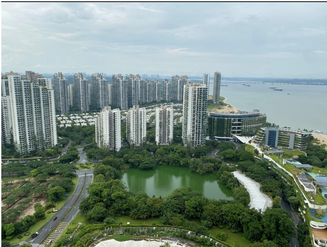
Fig 1: Forest City project in Tanjung Kupang, Iskandar Puteri
