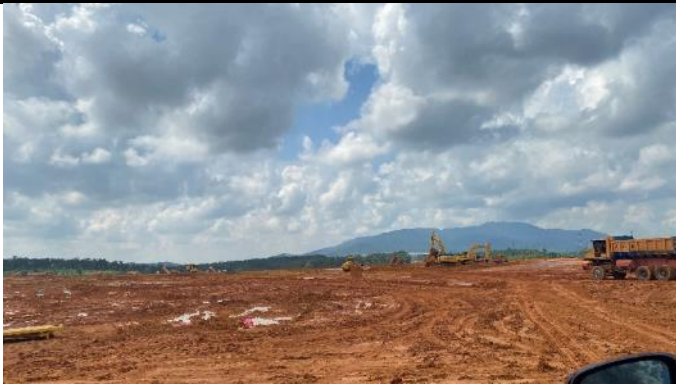
Fig 4: Ongoing earthworks at the site, 25 Sep 2024
