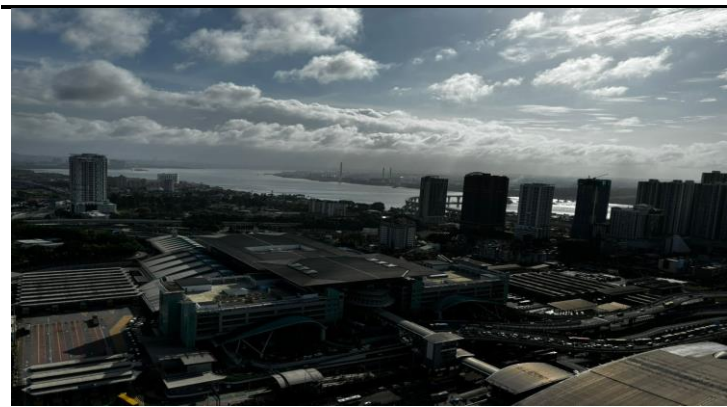
Fig 36: View of the CIQ being built
