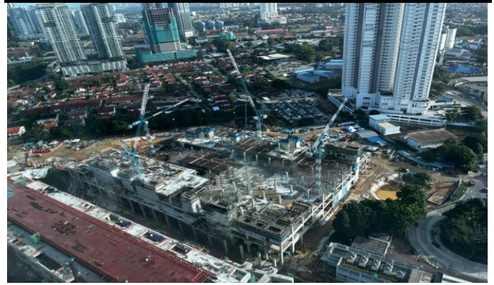
Fig 35: View of the RTS development from Menara JLand
