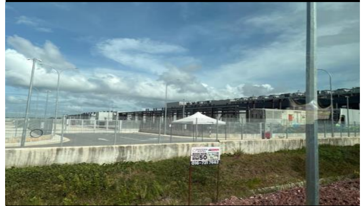
Fig 43: One that has received a CCC
