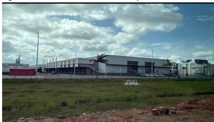
Fig 40: One of the first data centre to operate in Sedenak
