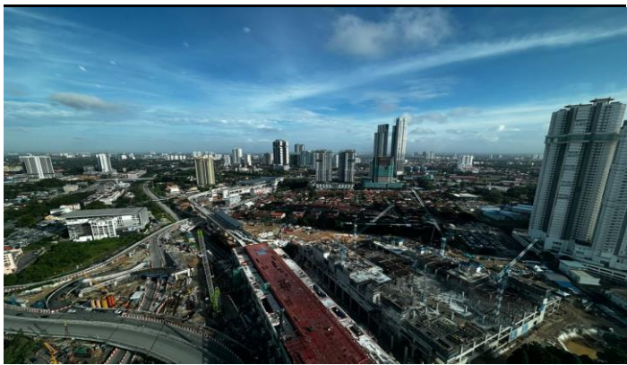
Fig 37: View of the RTS adjoining to Singapore and overseeing Senoko Power Plant
