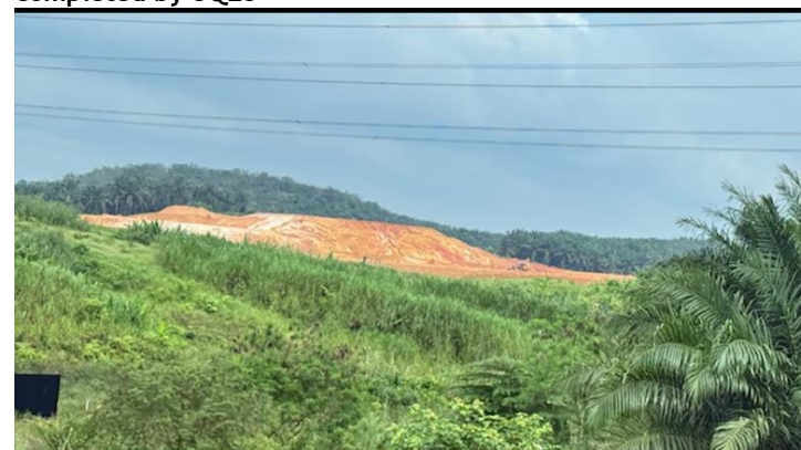
Fig 55: Earthworks at QUANTUM Edge business park will be completed by 3Q25
