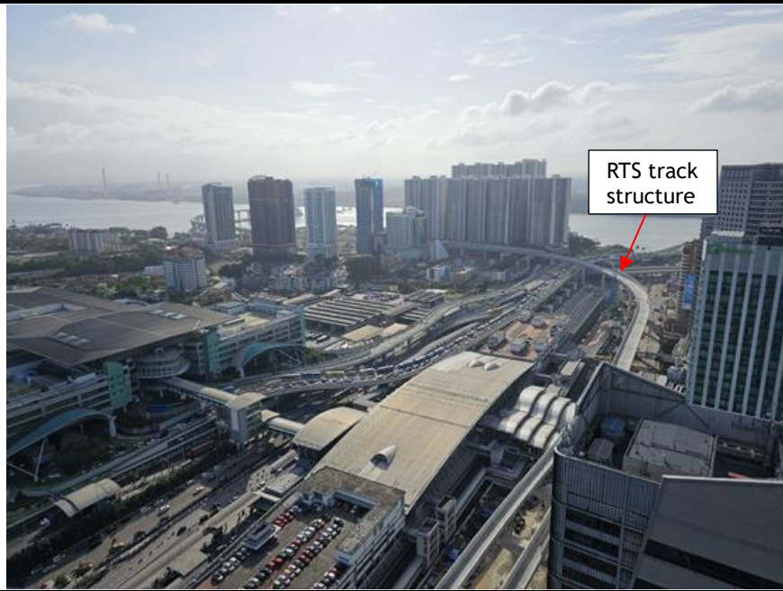
Fig 3: RTS Link Construction Progressing, On Track to Operate by Jan 2027
