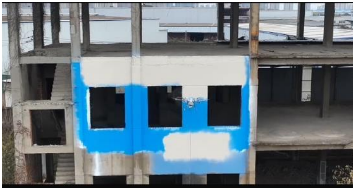
Fig 3: ISOTeam testing drone painting
