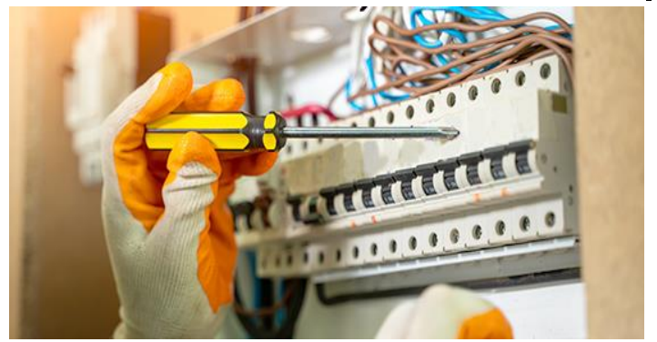
Fig 27: ISOTeam Homecare offers electrical work services too
