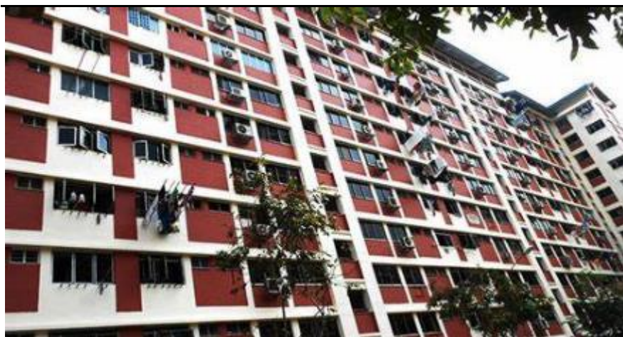
Fig 13: Repainting of the exterior of Bishan Street 22 by ISOTeam
