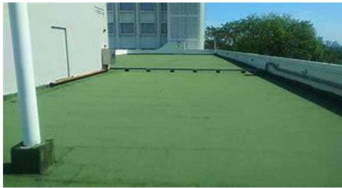
Fig 26: Green Label waterproofing membrane at NUS by ISOTeam
