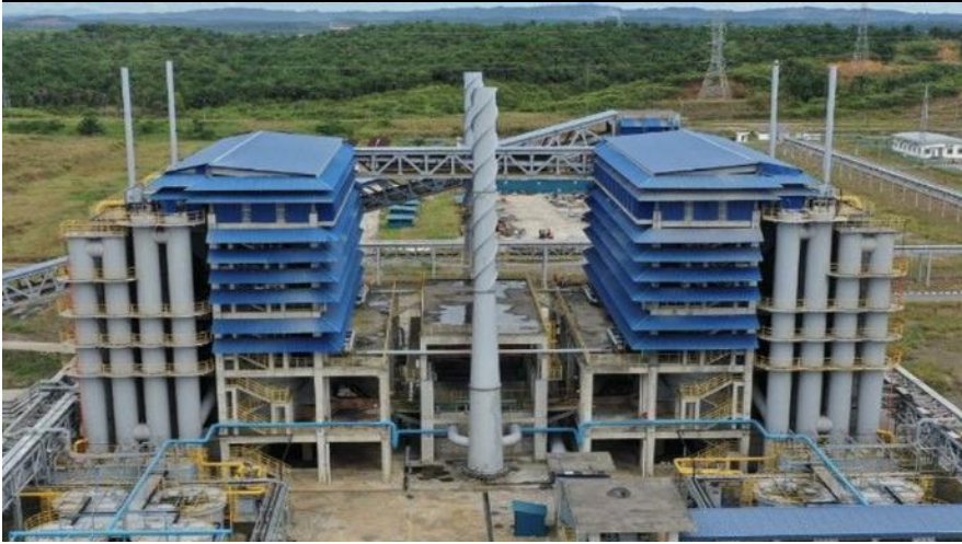
Figure 36: CMS phosphate plant (1)
