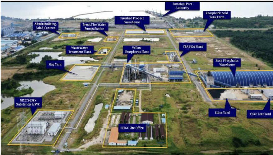
Figure 37: CMS phosphate plant (2)
