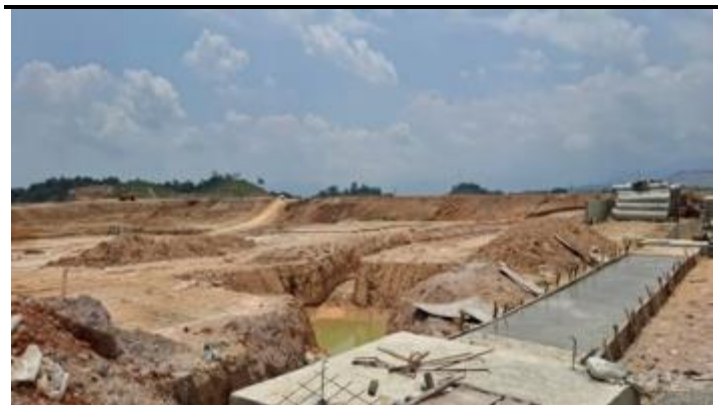
Figure 11: Earthworks at UMW HVM Park Precinct 5C (2)
