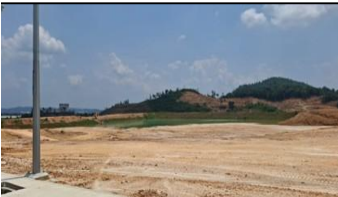
Figure 10: Earthworks at UMW HVM Park Precinct 5C (1)
