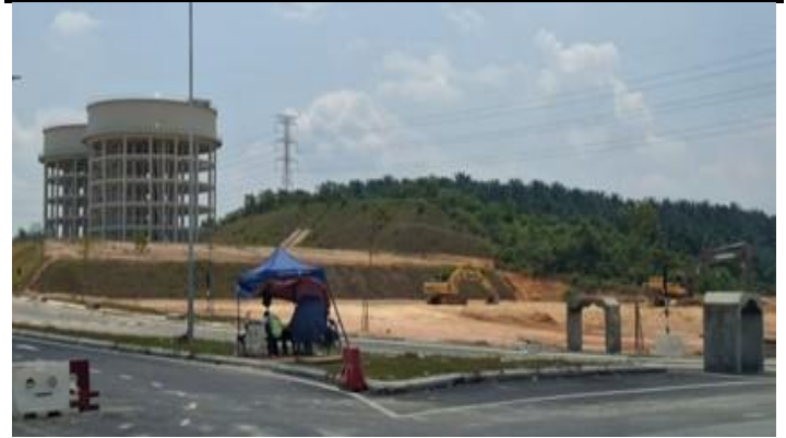
Figure 13: Earthworks at UMW HVM Park Precinct 5C (4)
