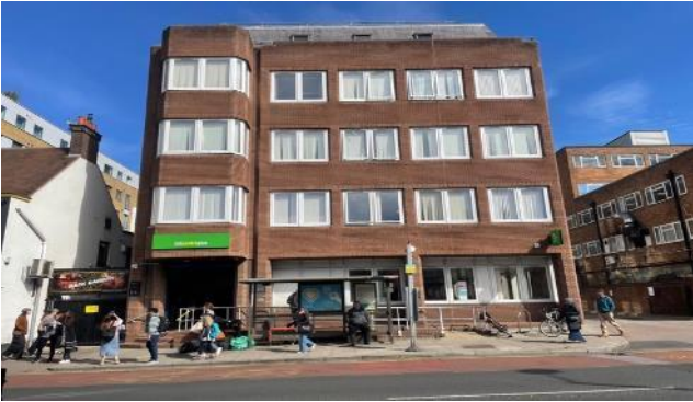
Fig 7: Broadway House, Jobcentre
