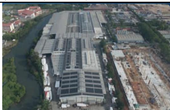
Fig 8: A bird's-eye view of the plant
