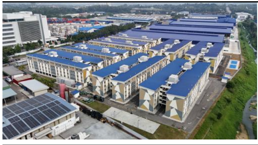
Fig 1: Worker accommodation asset in Pasir Gudang, Johor
