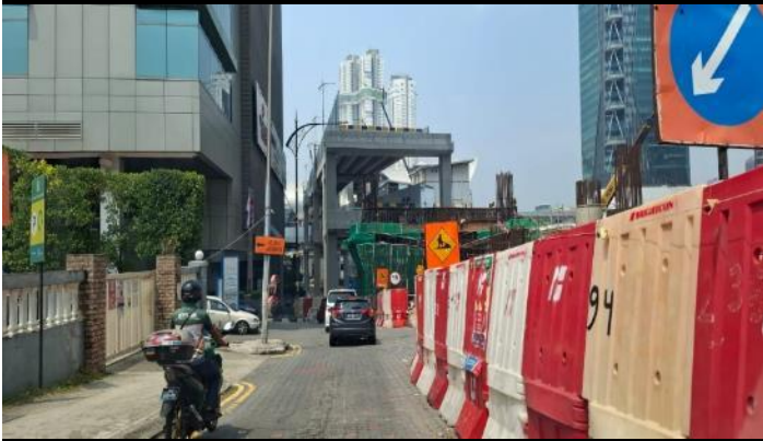
Figure 6: Flyover to Bukit Chagar station
