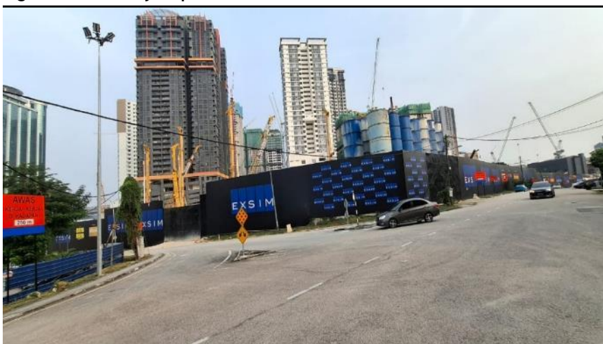
Figure 9: Causewayz Square construction site
