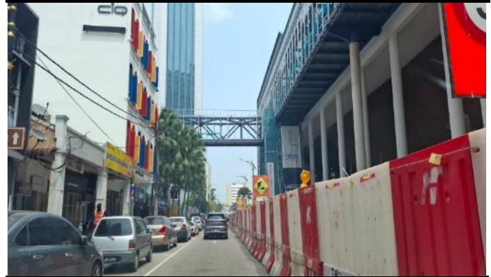
Figure 7: Pedestrian bridge to Bukit Chagar station
